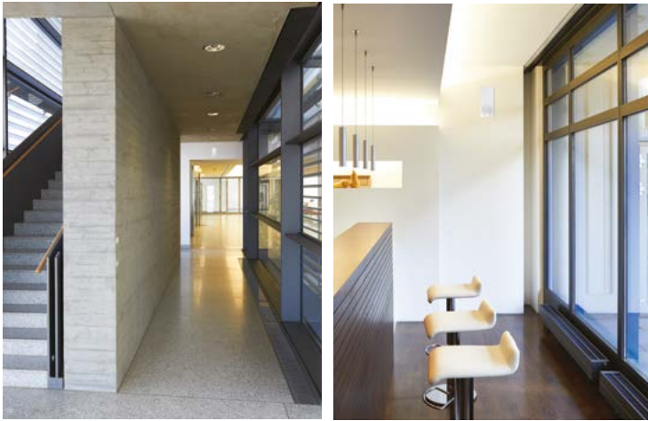
Typical flush mount applications - corridor and room with glass external wall.
